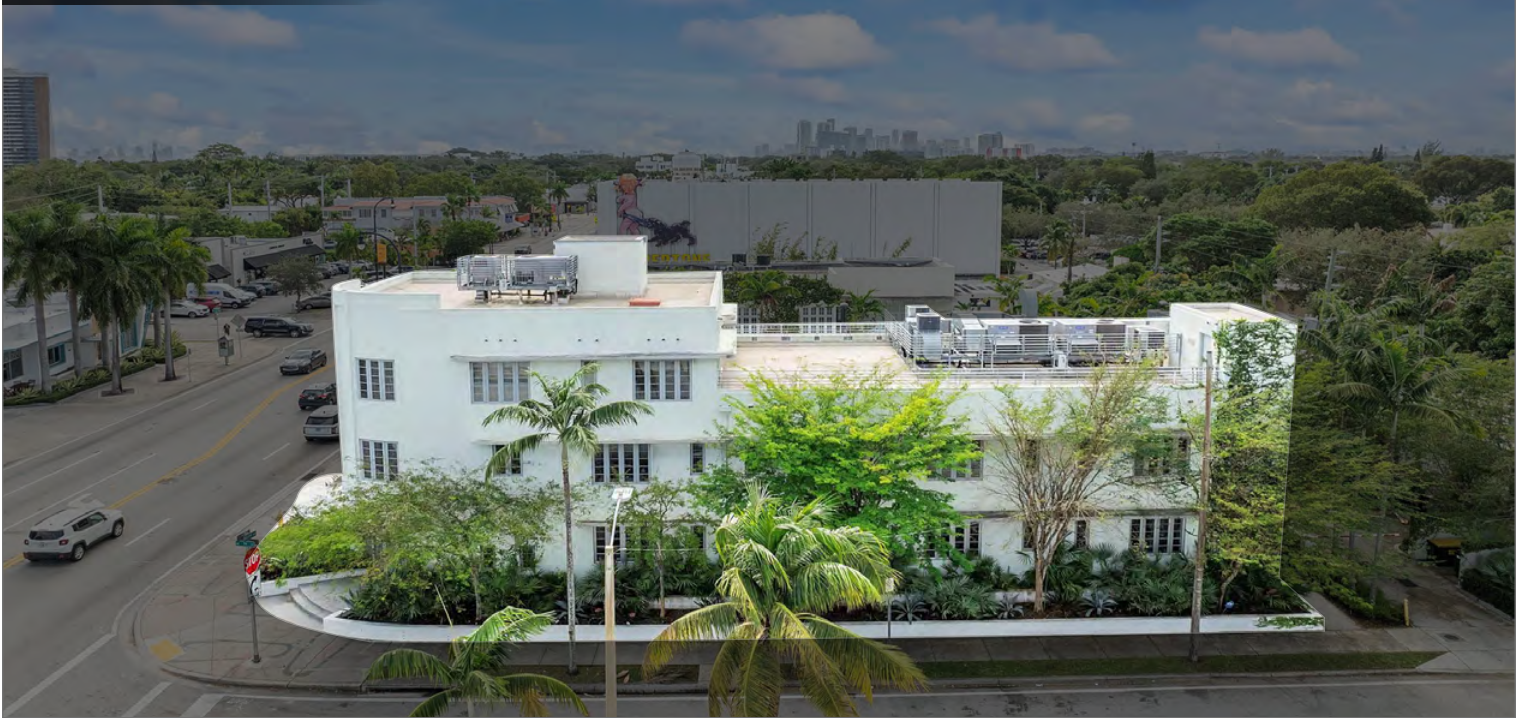
NORTH TO SOUTH VIEW
