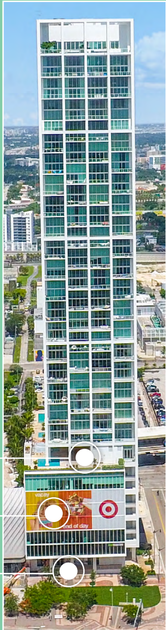
VIEW FACING EAST
